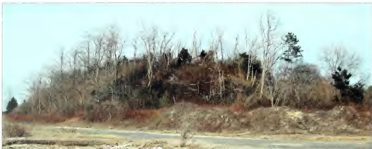
Figure 5.81. View looking northeast at the Battery Kingman engineered landform. This photograph shows the size and quantity of woody vegetation growing on Battery Kingman's engineered slope. All woody vegetation greater than four-inches diameter at breast height should be selectively removed to preserve the historic structure and its sheltering earthwork (Olmsted Center, January 2009).
